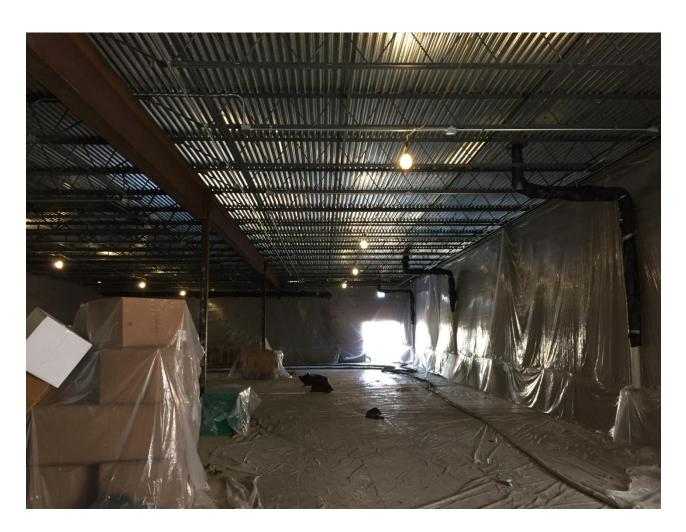
**WEIGHT ROOM –** The room is being prepared for installation of the sprayed on fireproofing of the steel structure.
