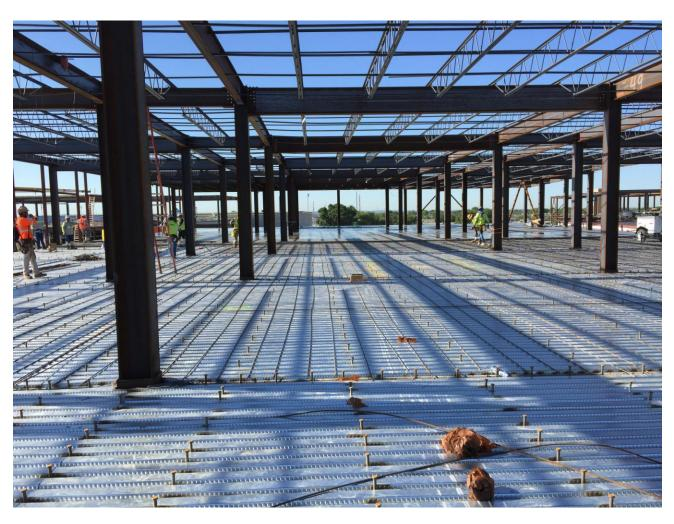
**CLASSROOMS** – The 3<sup>RD</sup> Floor of the classrooms adjacent to the PAC are being prepared for concrete to be poured. A portion of the floor beyond has been poured.
