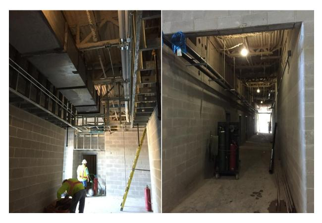
**ATHLETICS DEPARTMENT** – Metal stud framing for ceiling furr outs is being installed on the photograph on the left. Ductwork and above ceiling MEP work are in progress. The structural system above these spaces has received sprayed-on fire proofing.
