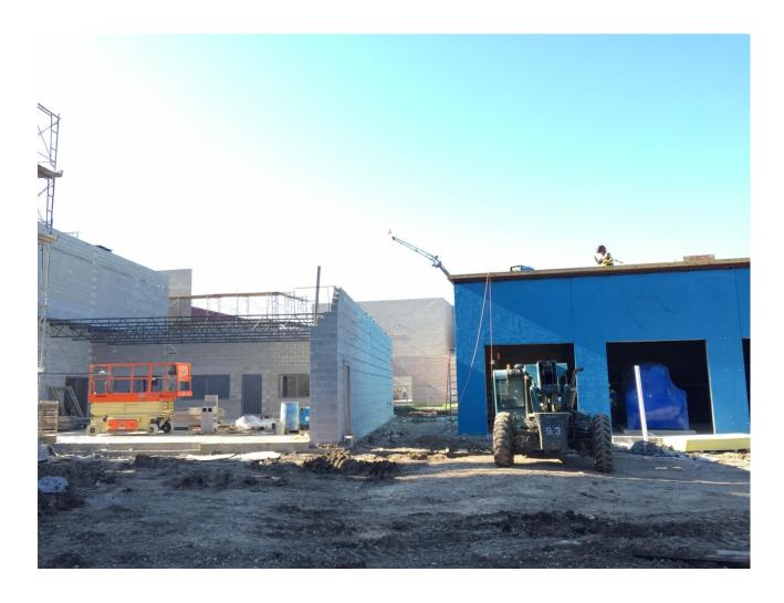
**MECHANICAL BUILDING & CONSTRUCTION LAB** – The small building on the right will house the mechanical equipment. The blue material on the surface of the block is dampproofing. Roofing work is in progress. The Construction Lab and Construction Classroom are on the left side of the photograph.
